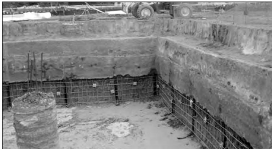
**Figure 1.26 Shotcrete and helical anchor shoring system**
